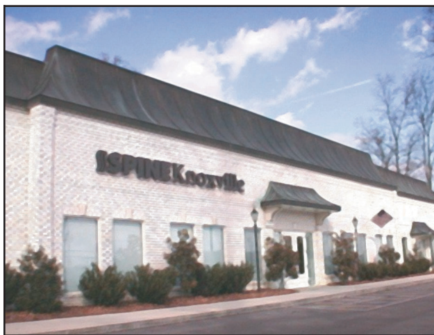
The SpineKnoxville facility in Knoxville, Tennessee.
